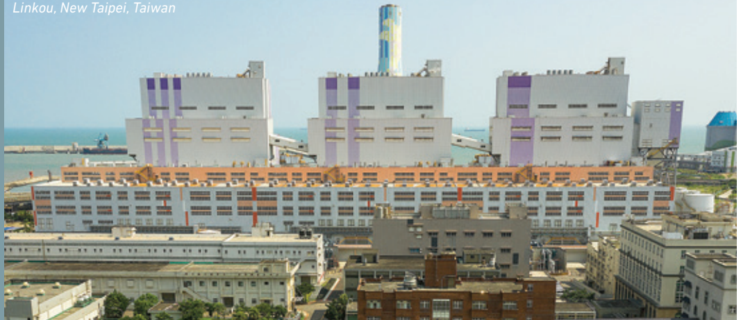
Linkou Power Plant Linkou, New Taipei, Taiwan
