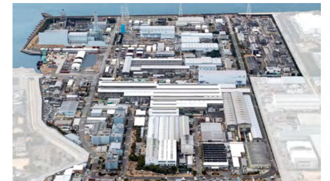
Takasago Machinery Works
