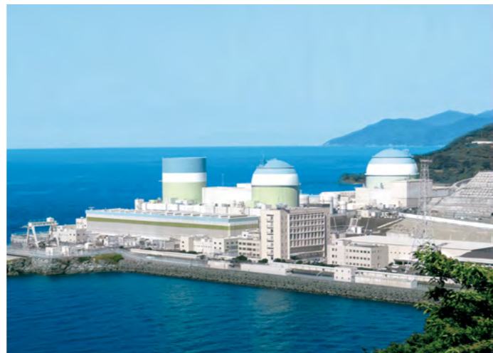
Ikata Nuclear Power Plant
