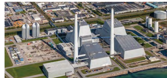
Example of Biomass Plant Denmark/Avedøre #1/250MWe
